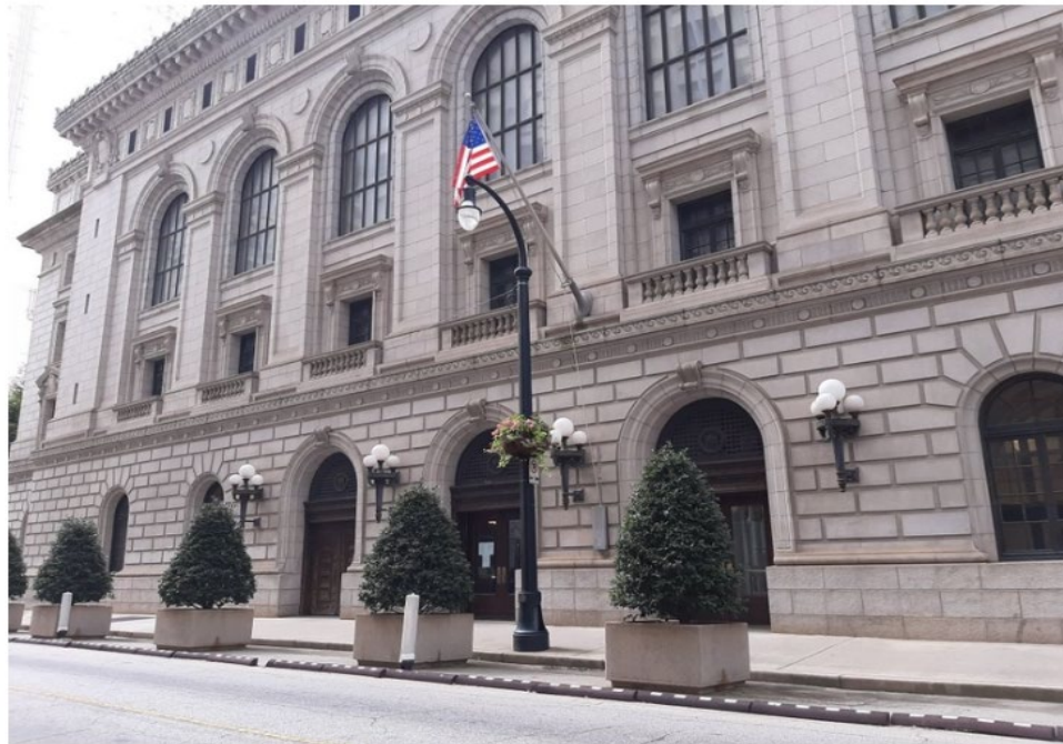
Elbert P. Tuttle Courthouse in downtown Atlanta, home of the U.S. Court of Appeals for the Eleventh Circuit. (Photo by John McCosh/Georgia Recorder)
